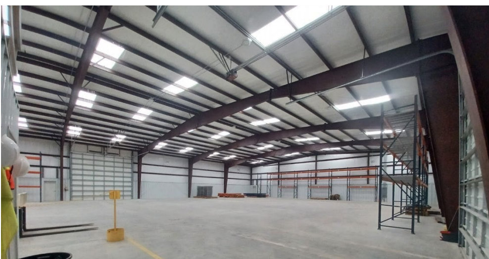
RACKS ARE AVAILABLE
