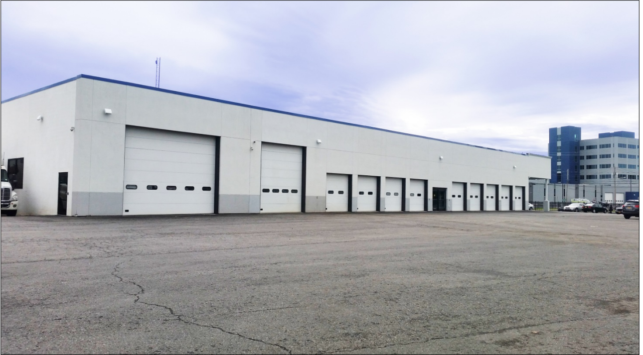
North Side of Building with 11 Grade-Level Overhead Doors
