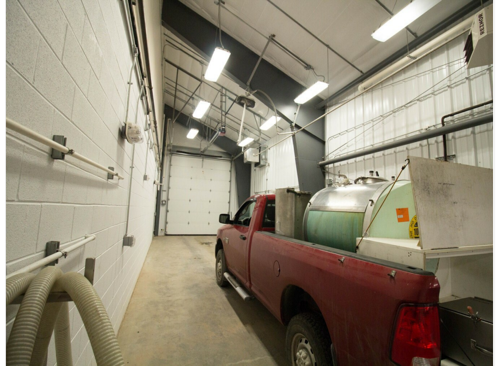
Truck loading bay and receiving
