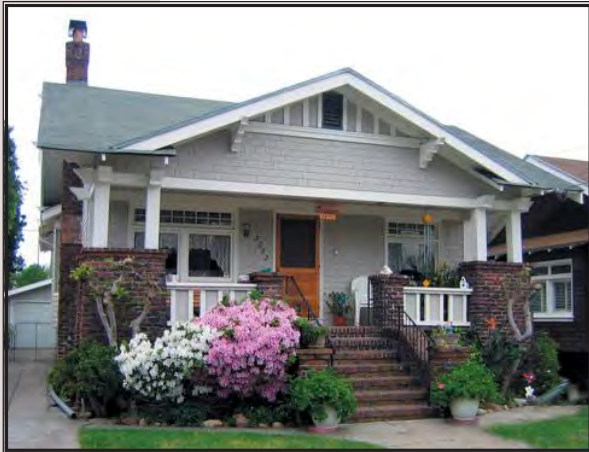
EXPOSED RAFTER TAILS AND TRIANGULAR KNEE BRACES ARE COMMON ELEMENTS OF THE EXISTING NEIGHBORHOOD
