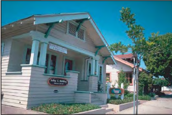
PROVIDES PROFESSIONAL OFFICES IN FORMER RESIDENTIAL BUILDINGS
