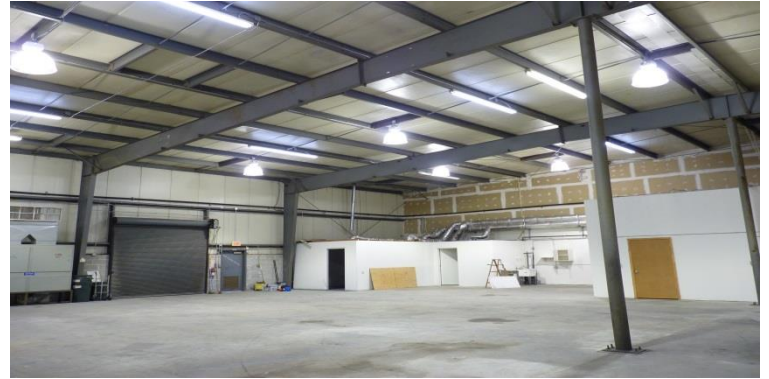
AMPLE LIGHTING IN WAREHOUSE, 10' X 10'
