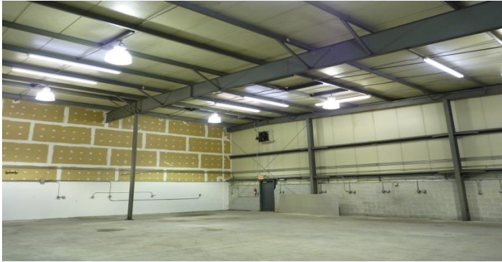
POWER DISTRIBUTED AROUND EXTERIOR WALLS OF WAREHOUSE, 17'-19' CLEAR, FREE SPAN
