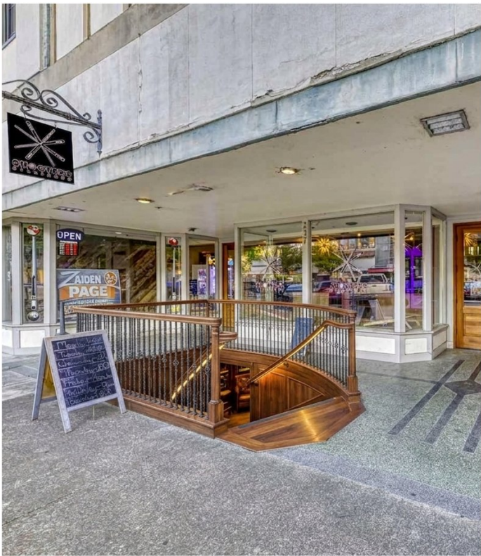
Wood framing in place for cellar stair installation. Staircase shown is a rendering.
