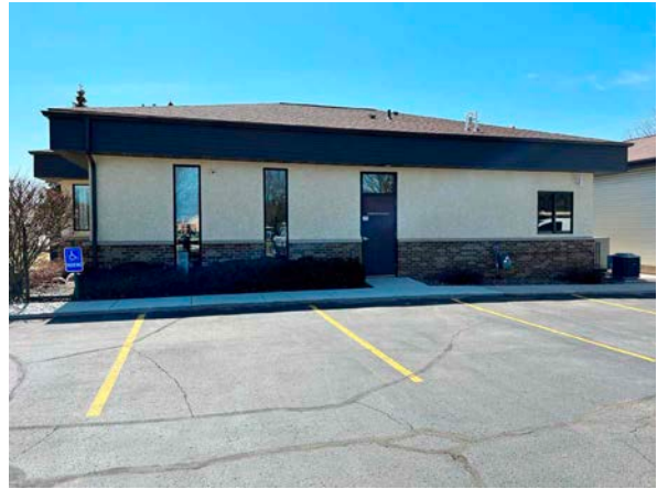
Side (North) Entrance
