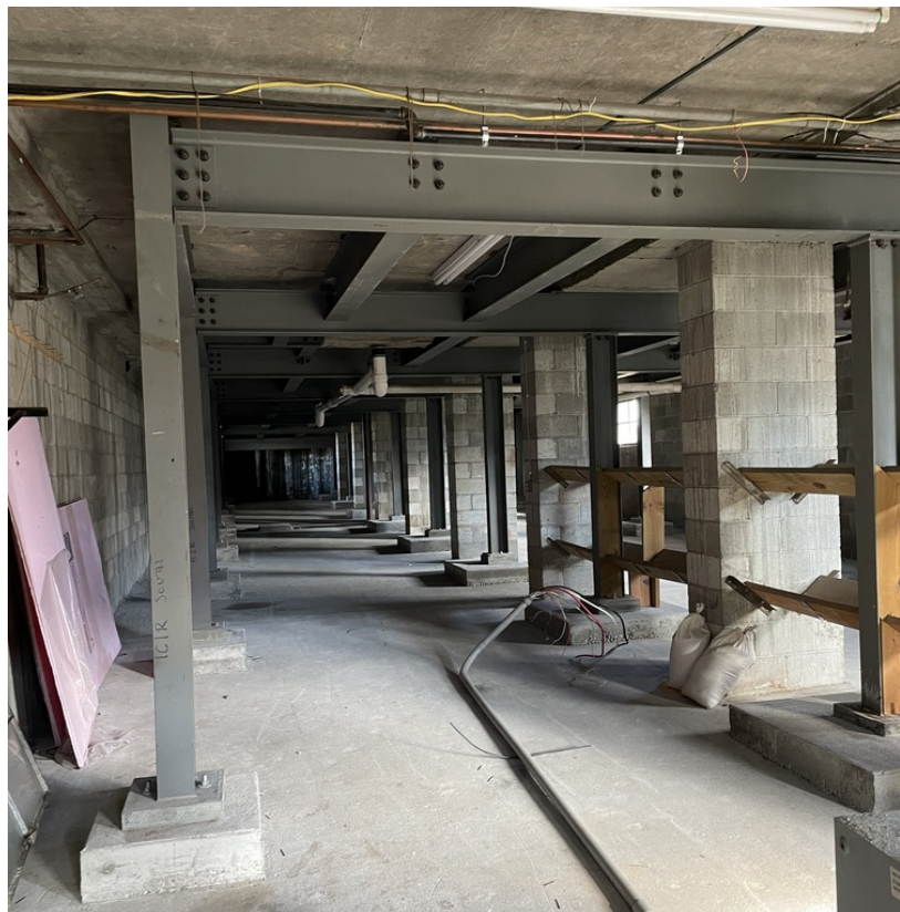
Basement provides additional storage space
