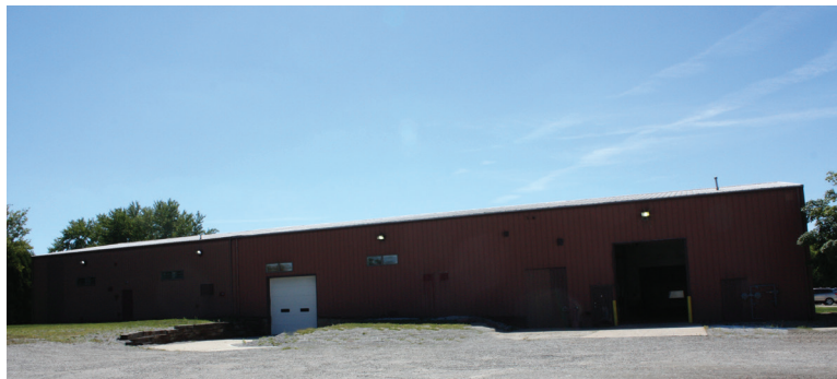
BACK OF BUILDING
