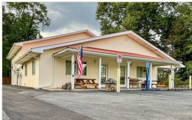
Front exterior view
