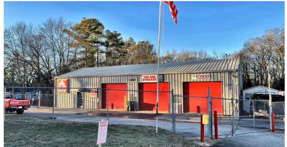
Lexington Road frontage and secured storage yard
