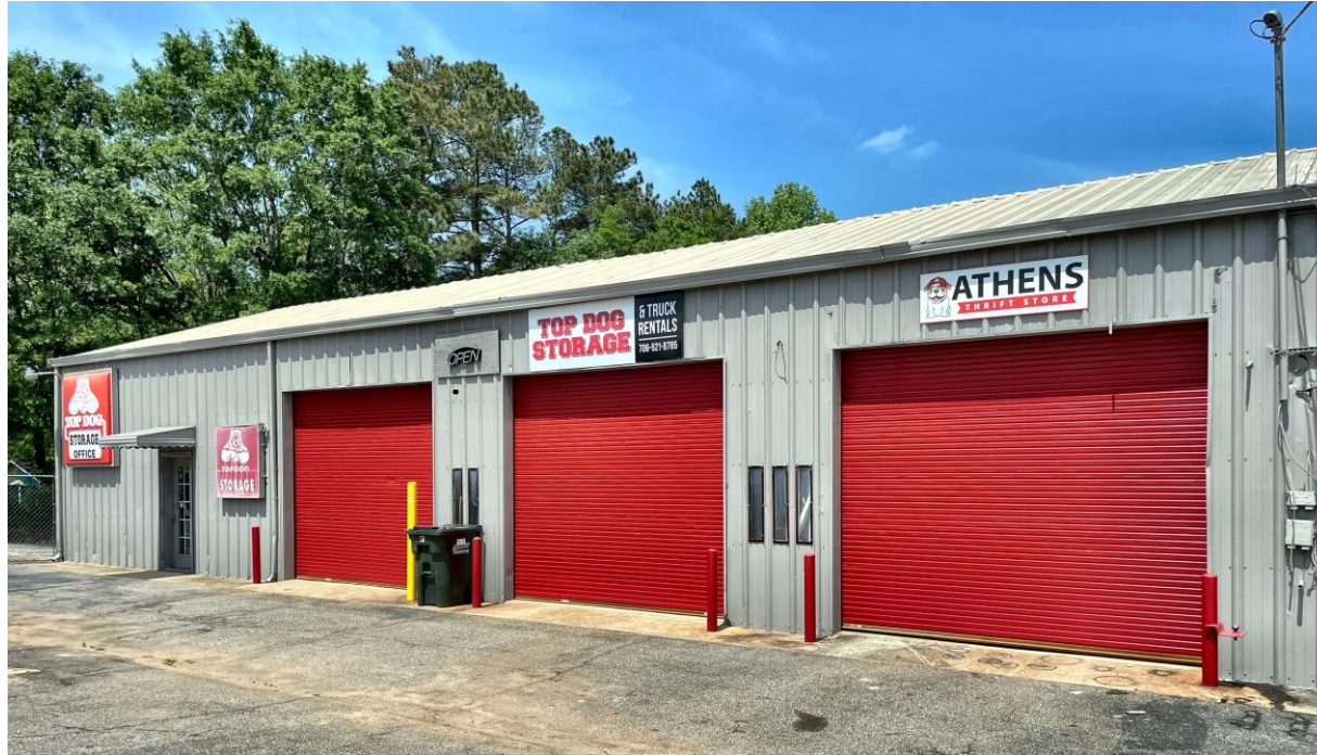
Lexington Road frontage — drive-in overhead doors
