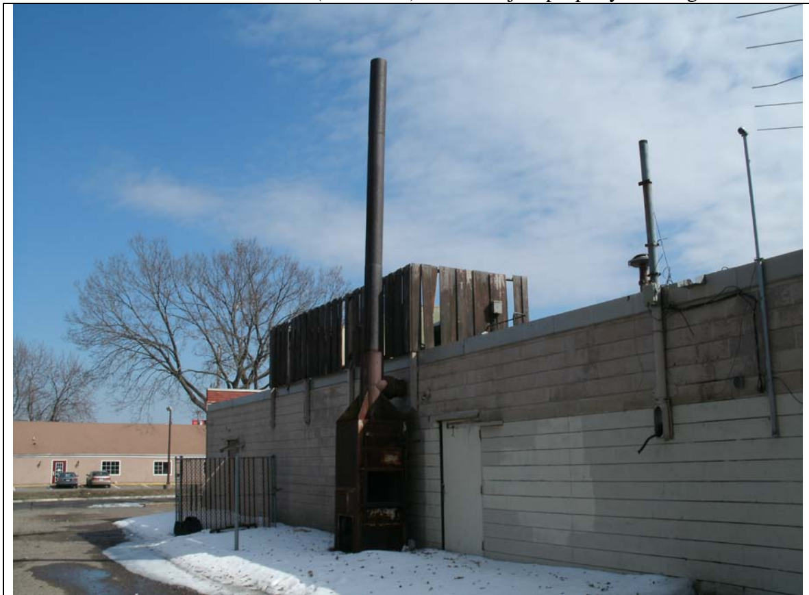
Photo #2 Backside of the subject property building.
