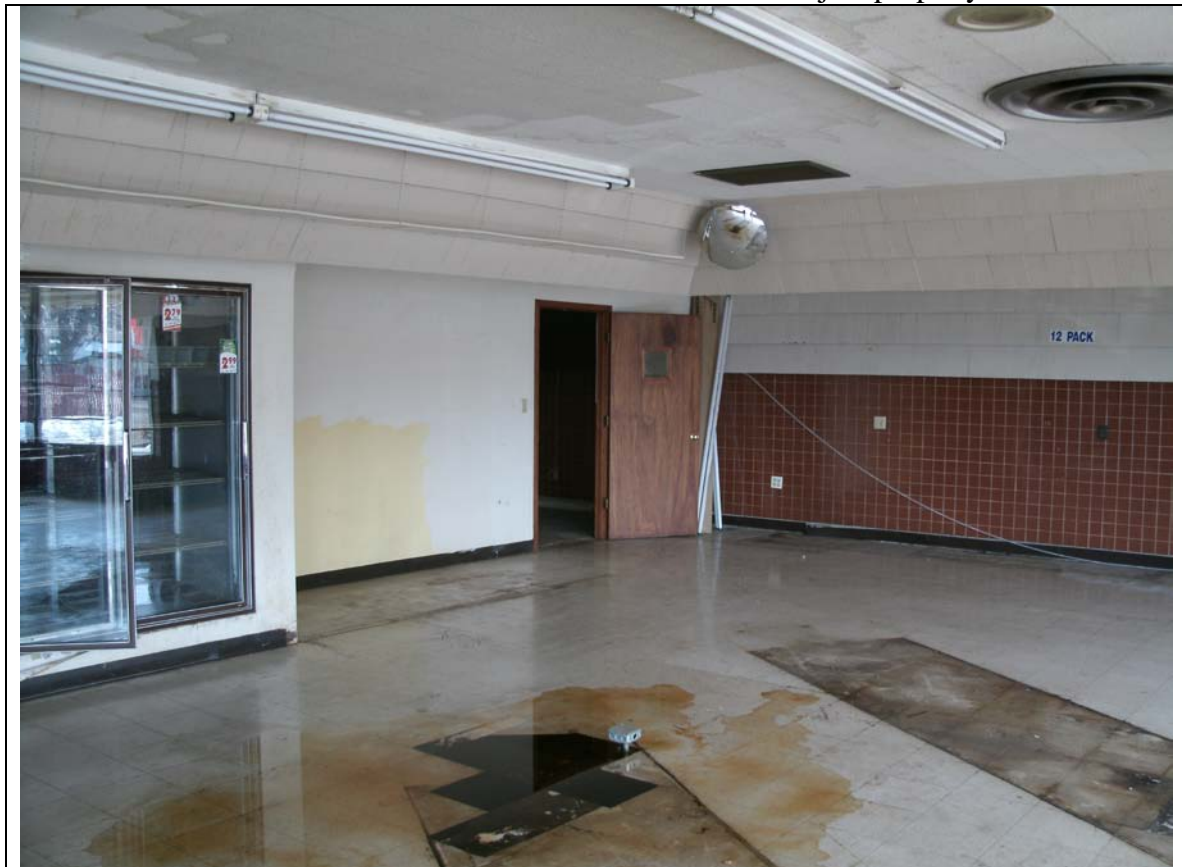
Photo #4 Typical interior conditions of subject property building.
